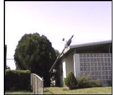
Move Up the Roof as you Pull the Collector Up a Foot or so at a Time.
